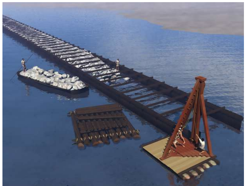
The construction of dikes to channel «Aude» at Mandirac © P. Cervellin, CNRS
